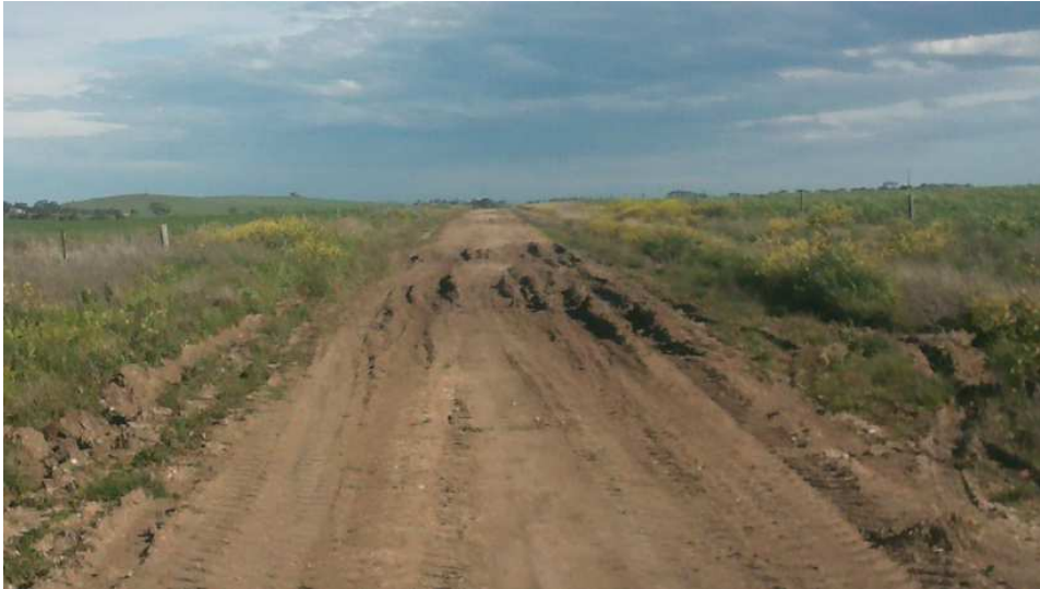
Typical Class 4b Rural Sheeted Road in wet conditions
