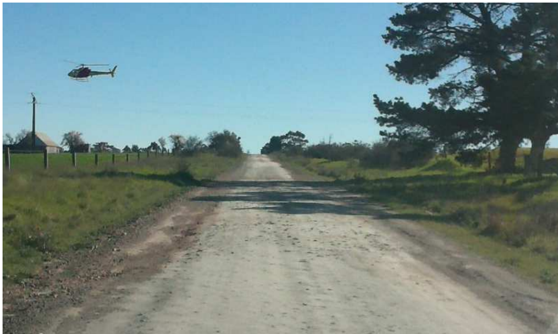
Typical Class 2a Rural Sheeted Road approaching CEoL
