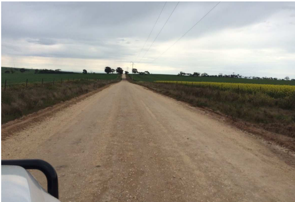
Typical Class 1 Rural Sheeted Road in fair condition
