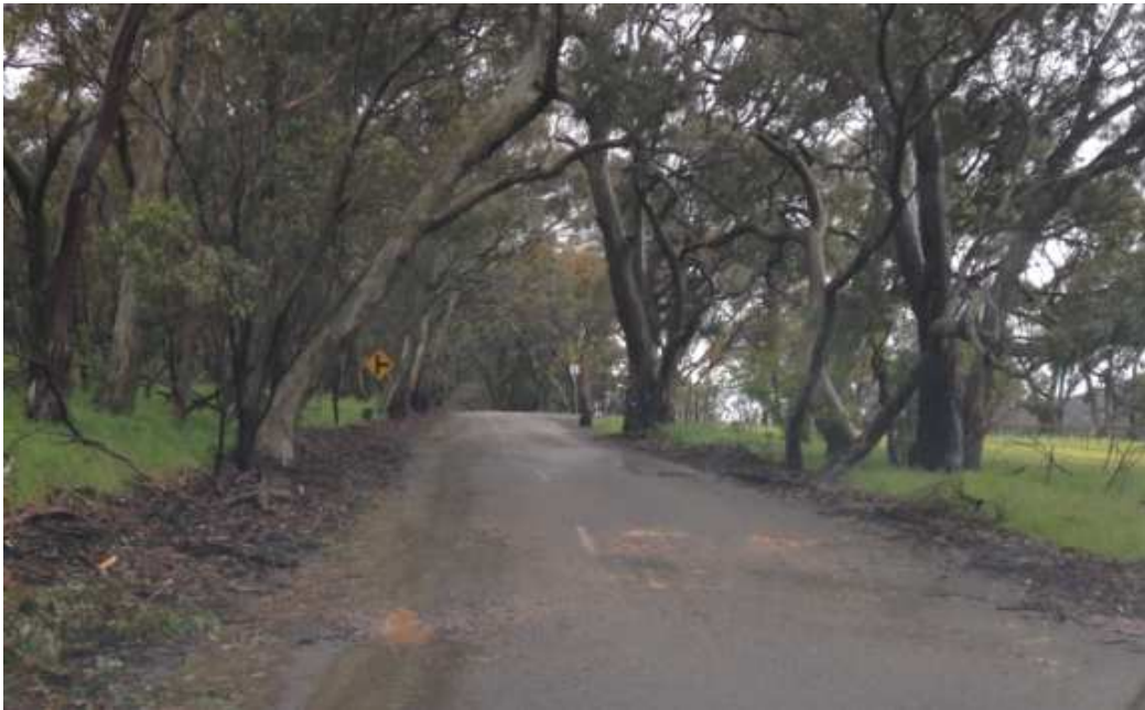
Typical Rural narrow road seal
